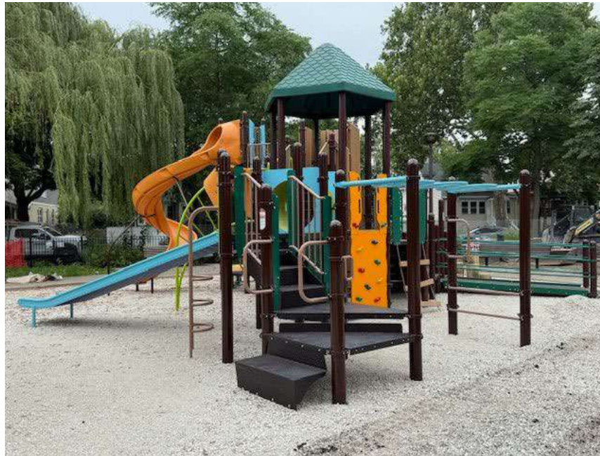
Andersen Park renovation
