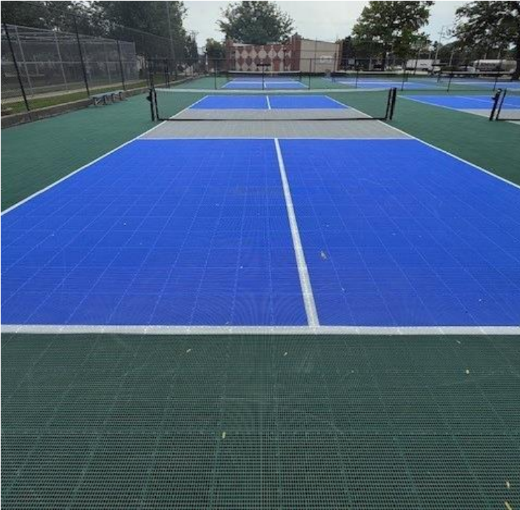
Retrofit with tiles for Pickleball surface
