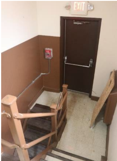
South stair and basement under kitchen
