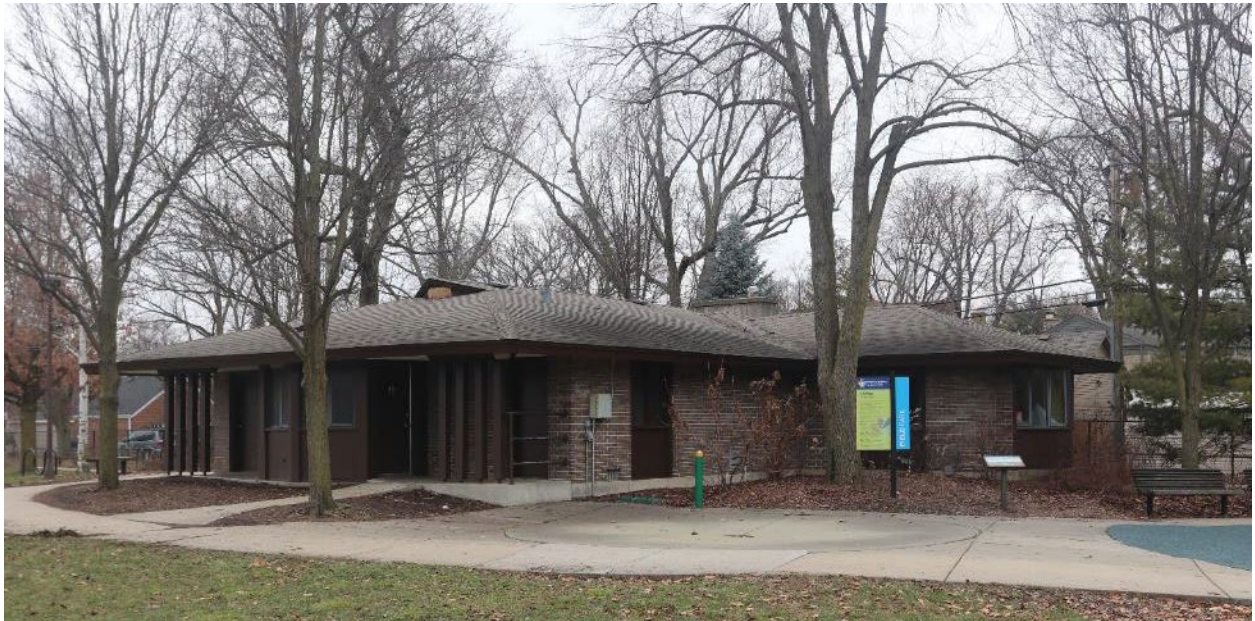
View of Existing Center from Northeast across Splash Pad
