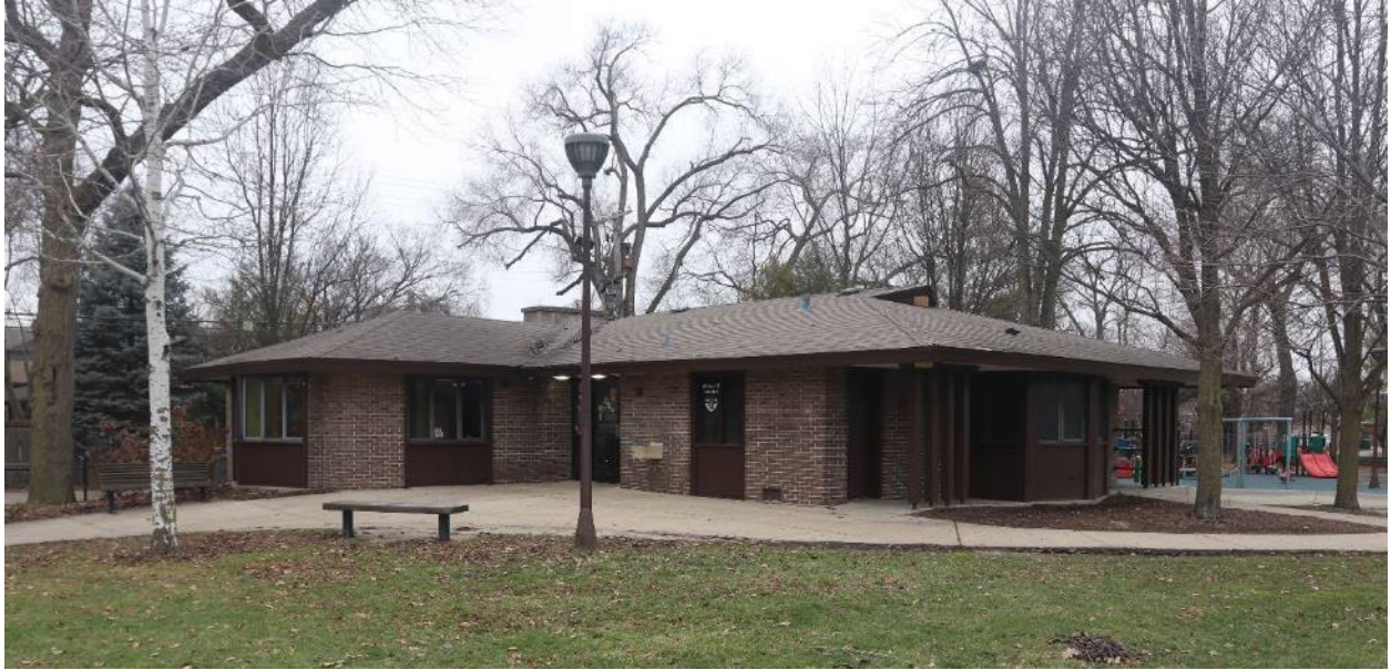
View of Existing Center from Southeast to Main Entry
