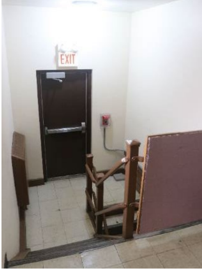
North stair and north basement
