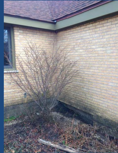
Drainage and damp issues
